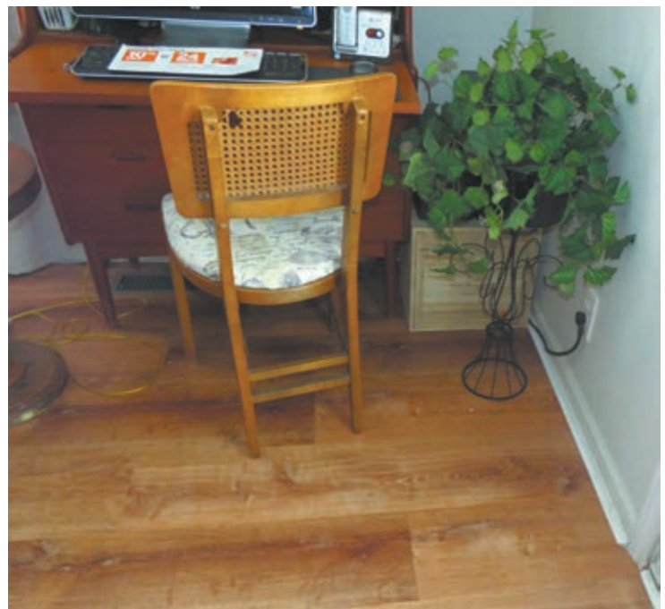
By taking up worn, wrinkled carpet and replacing with vinyl laminate flooring, a serious trip-hazard is corrected.
