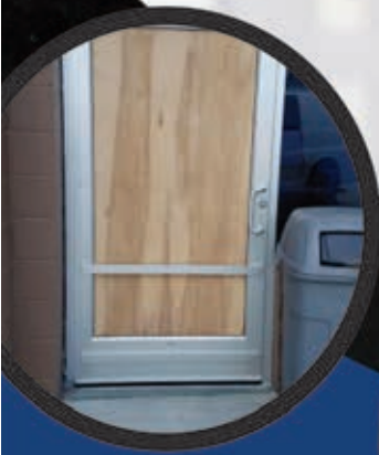
Board Ups & Glass Replacement
